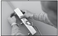
The flange of the clamp must be hooked under the seam before the bolts are tightened.
