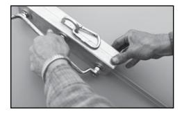
Once the clamp is hooked under the seam, over a clip that is fastened down, tighten the bolts with a ¾-inch, box-end wrench.
